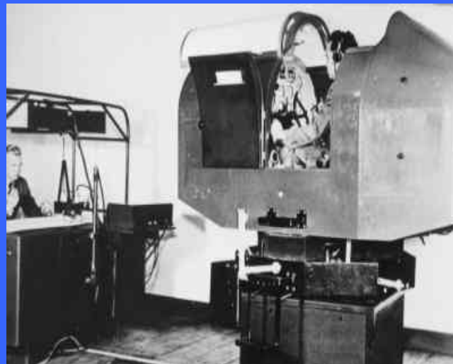
1930 - Link trainer (pneumatic platform)
