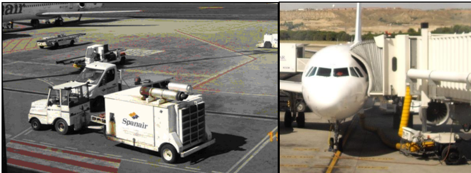
Figure 2.15 ACU (left) and ACU built in the passenger bridge (yellow hose in the right picture)
