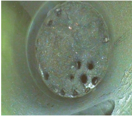
An oil-contaminated air duct and air outlet, Boeing 757 (Iceland Air)
